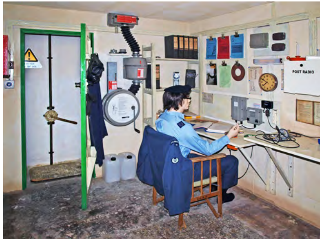
This is a general view of the recreated monitoring room, looking toward the shaft and toilet in 2014. The door shows Fred's deflector modification, the sump pump is visible beyond. On the wall is the Luwa filter system, shown in its 'Active' condition – 'Pete' enjoys a cigarette! The post radio was never issued to Catforth but is displayed in the correct location.
